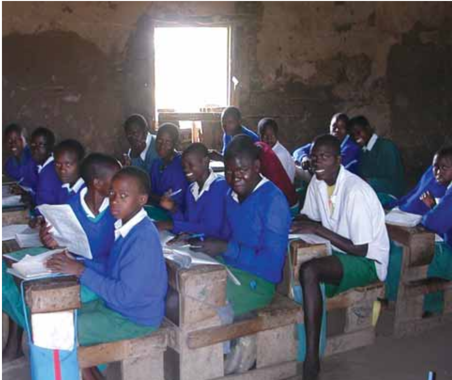
This is an elementary classroom with students from the Mara Region of Kenya. It is an old classroom with dirt floors and walls of mud/dung/sticks with a single window with no glass. Martin Herbst's students worked on construction of a new school to replace classrooms like this. (Photo by Martin Herbst)
